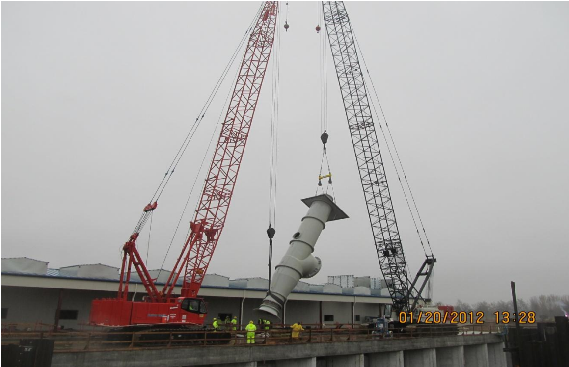
Balfour Beatty picking 84" pump to vertical position using two cranes.
