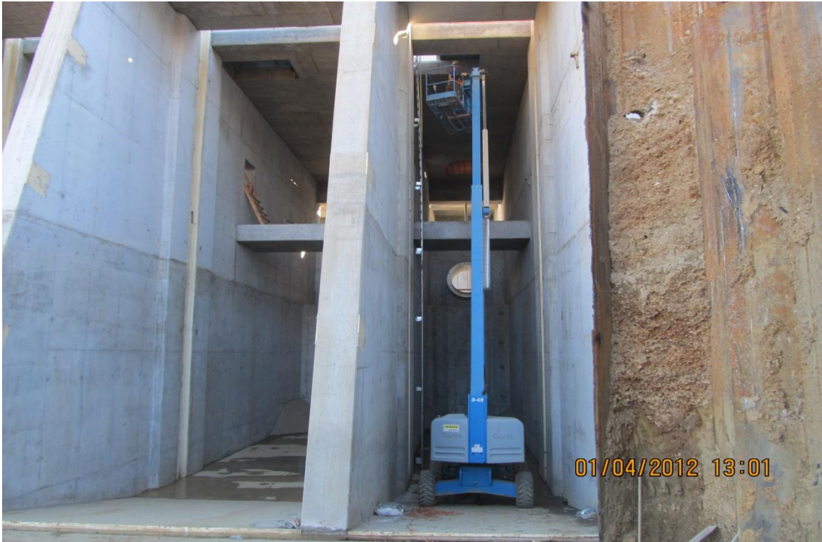
Balfour Beatty carpenters installing sump access ladders on the sump wall.
