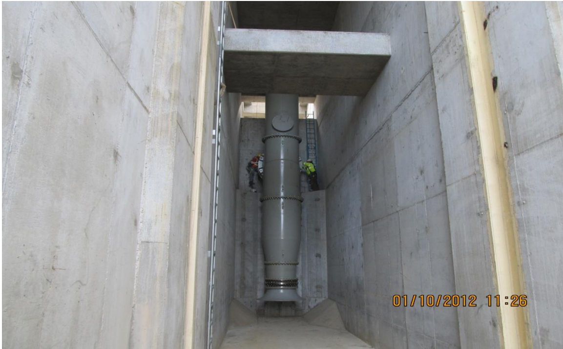
Balfour Beatty connecting 60" pump to the discharge pipe.
