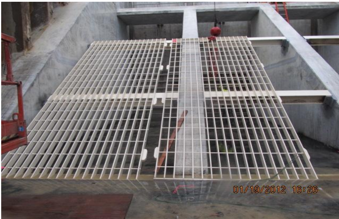
Balfour Beatty installing siphon intake trash racks.
