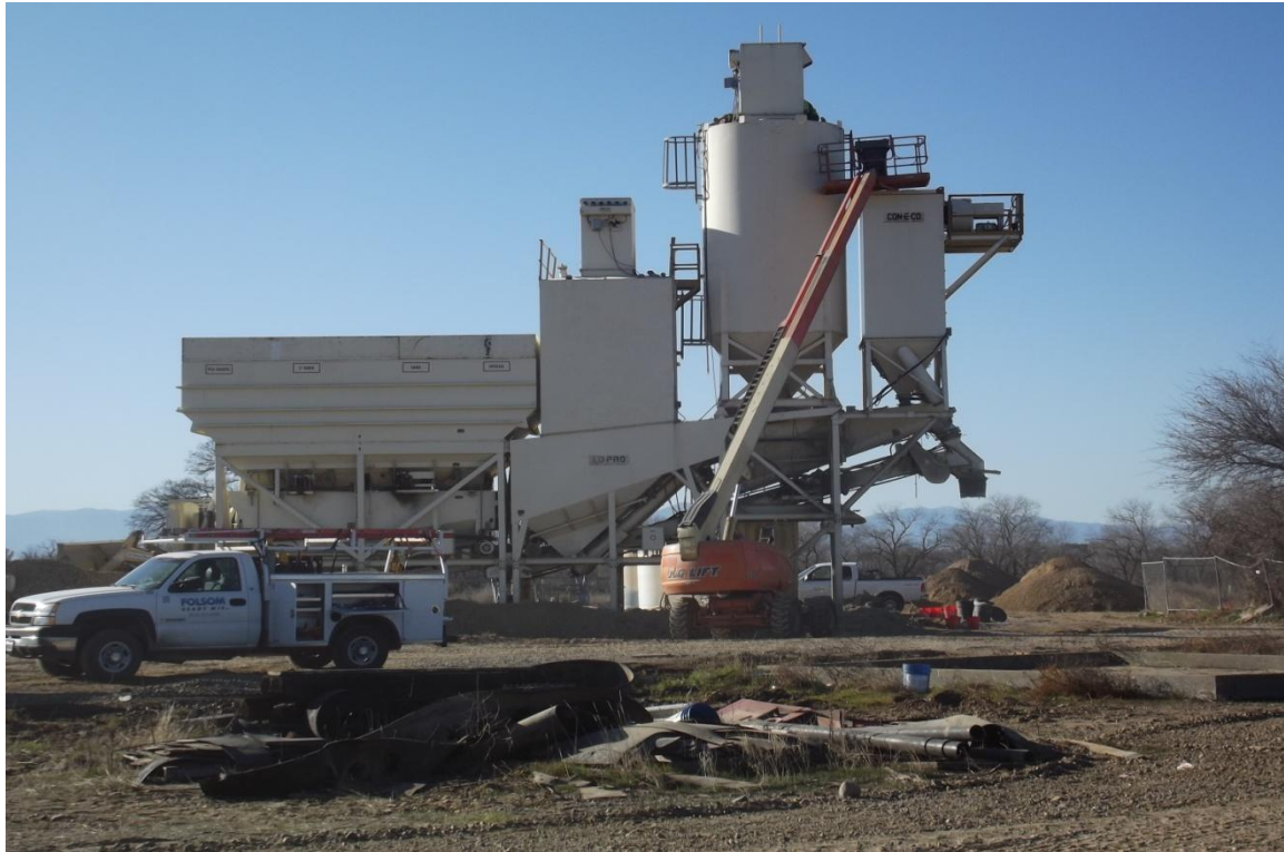
West Bay Builders subcontractor Folsom Ready Mix disassembling the batch plant.
