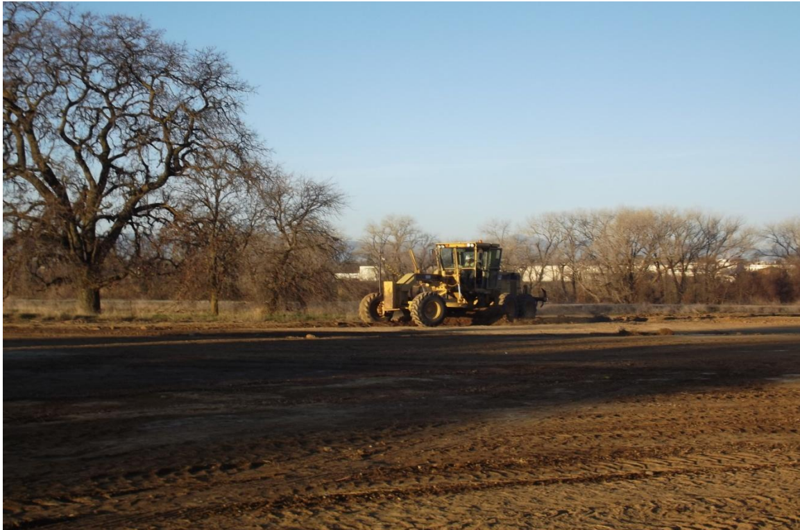
West Bay Builders subcontractor Meyers grading staging area to final grade.
