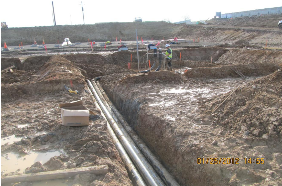
Balfour Beatty installing 5" conduit trench from switchyard transformer pads.
